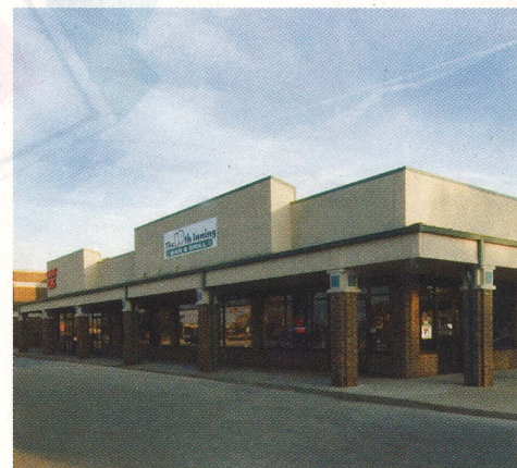
Paul Hemmer Cos. recently acquired the 87,000-square-foot Riverside Pavilion in Rockford, Ill., for $6.8 million.
