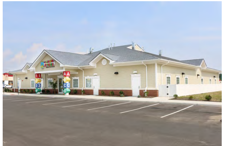
The Learning Experience 10,000 square foot building
